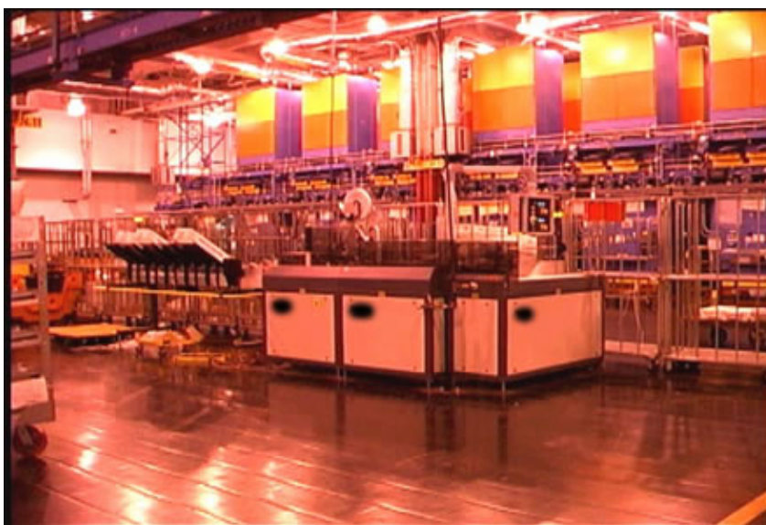
Tabbing system on plant floor at a Processing and Distribution Center
