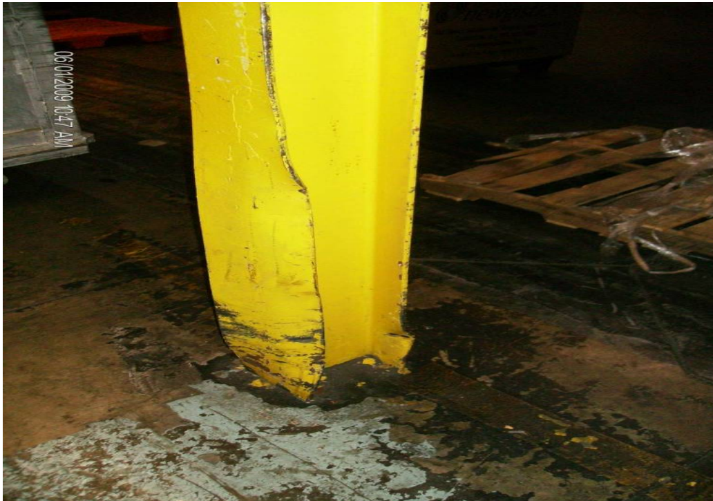
Illustration 5: Severe damage to a supporting column caused by a vehicle impact.
