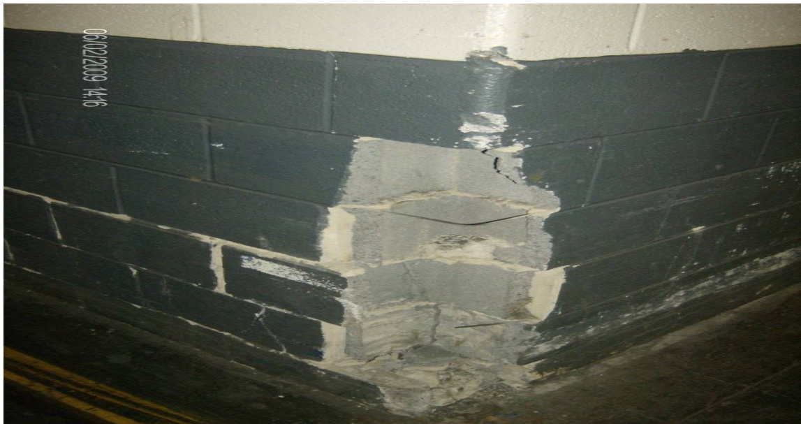
Illustration 7: Damage to a building from a vehicle impact.
