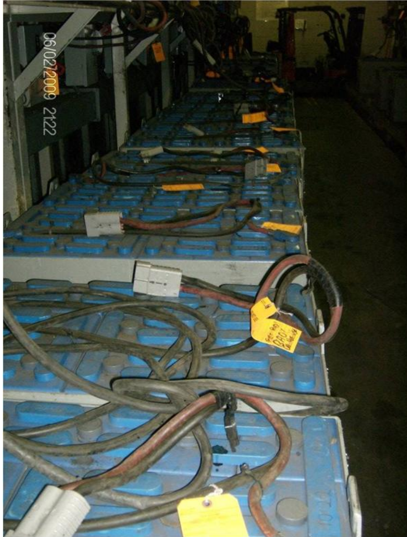
Illustration 11. Batteries labeled with tags were not functioning properly.
