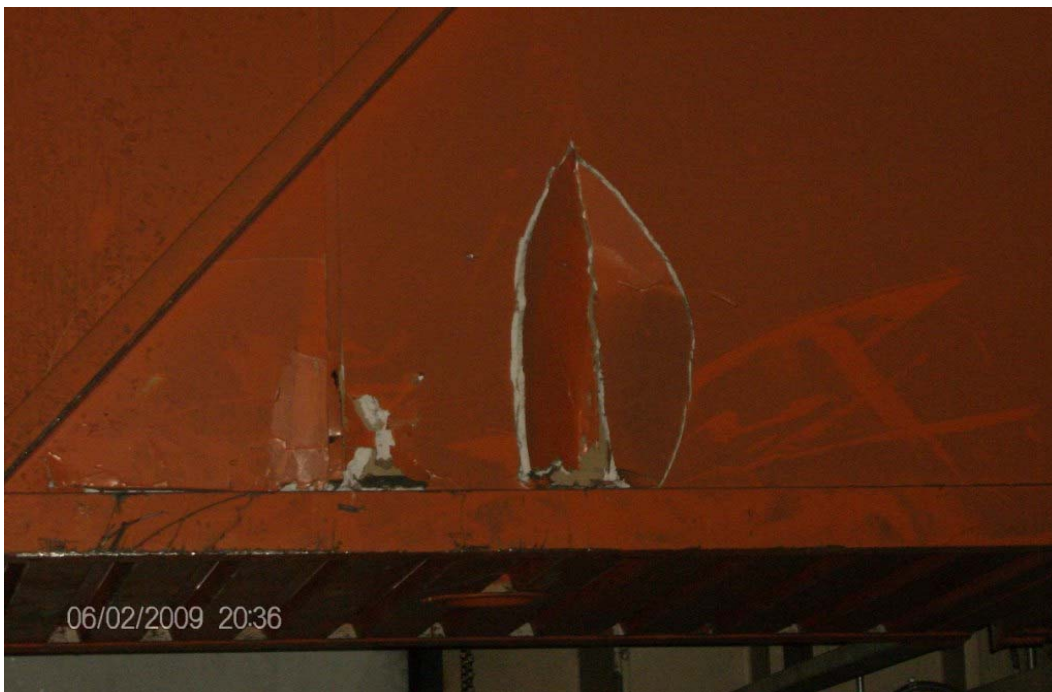
Illustration 6: Damage to an overhead look out gallery caused by a forklift with the mast raised.
