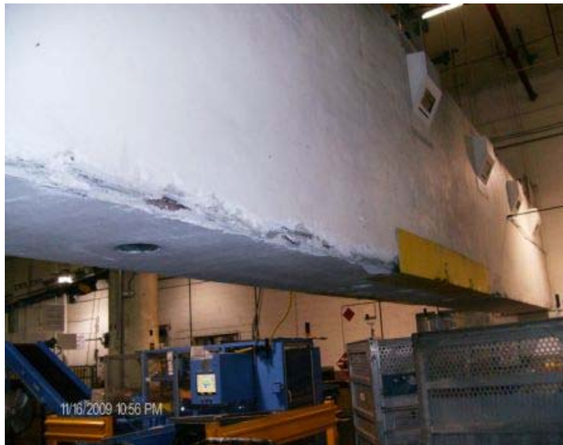
Illustration 6: Damage to the observation area at Grid G9, Indianapolis P&DC, 11/16/2009.
