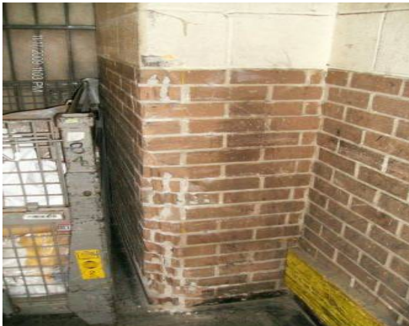
Illustration 7: Damage to brick corner near Bay 25, Indianapolis P&DC, 11/17/2009.
