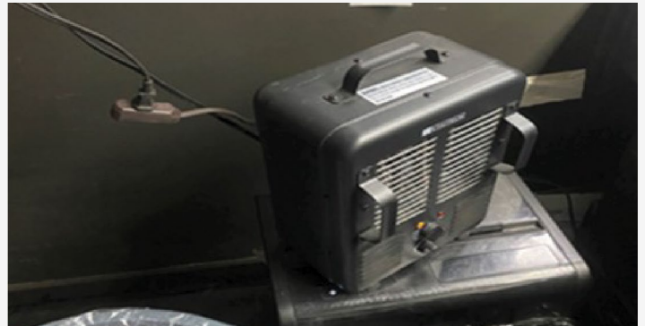
Figure 3. Portable Heater Plugged into an Extension Cord
